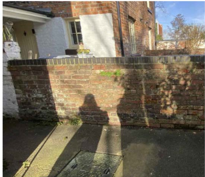
4 Typical Coping Detail to party walls NTS
